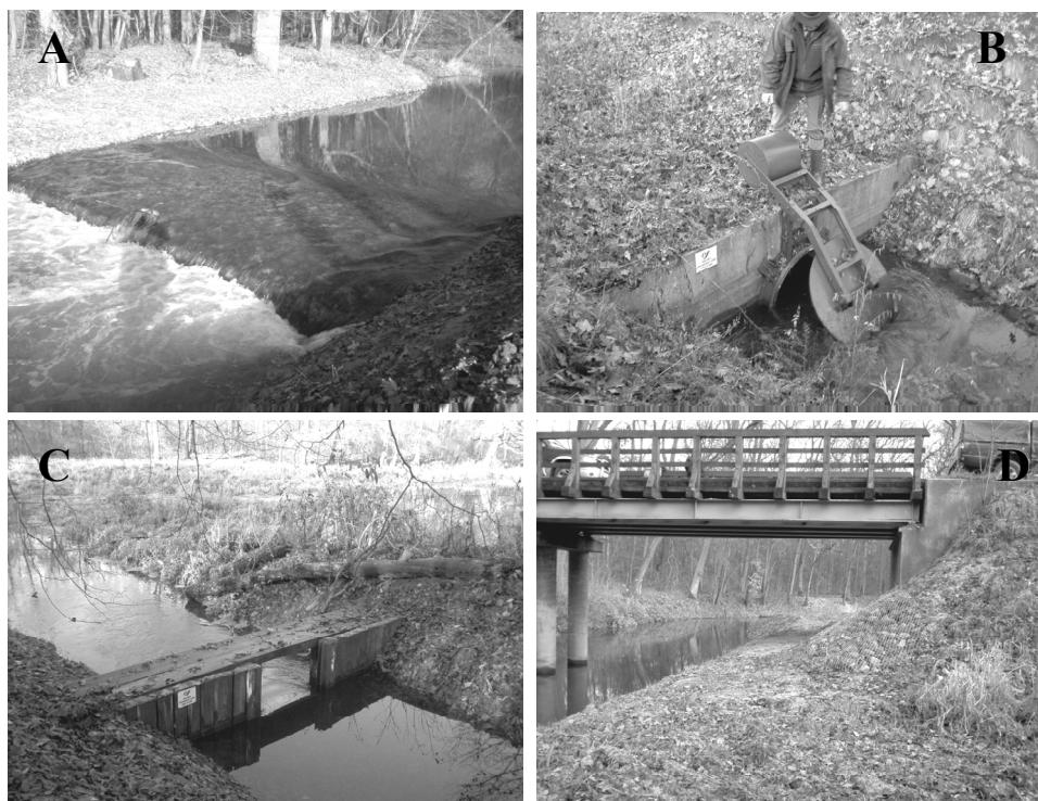
**Figure 4.** A damming sill (A), a culvert with a flap check valve (B), a log stop gate (C), a bridge on the Lutynia River (D)
