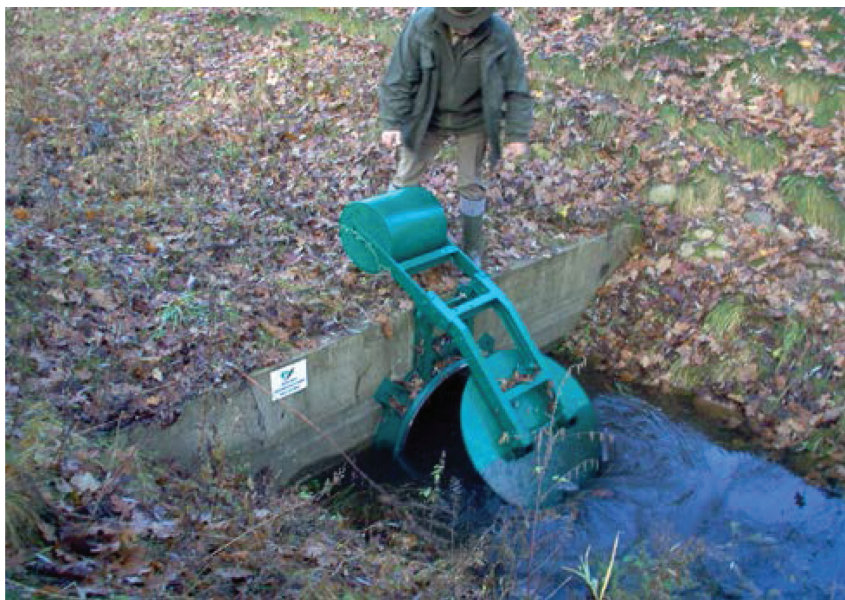
Figure. 3. A culvert with a backwater valve gate
