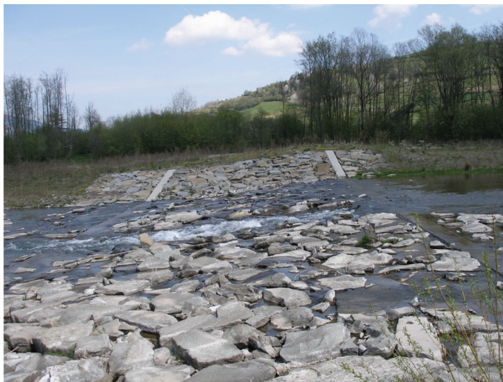
Photo 1. The bloc ramp on Porebianka stream – please notice curtain walls, photo A.Radecki-Pawlik
