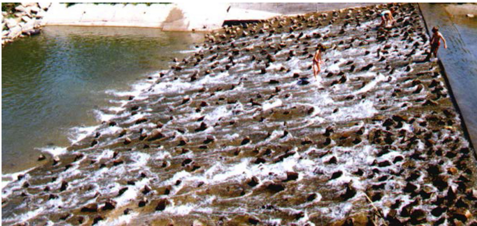
Photo 3. The bloc ramp on the Brennica river, photo. A.Radecki-Pawlik
