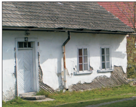
Phot. 45. A fragment of a wooden house with the ground floor almost at the ground level: walls plastered with clay laid on wooden slats; the entrance door covered with decoratively arranged clapboards and a transom window (photo: W. Bieda)
