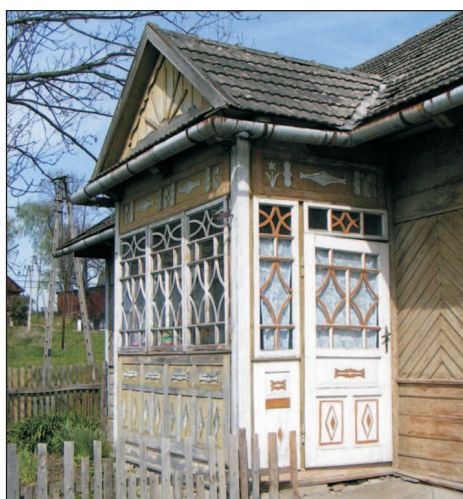
Phot. 56. A closed porch with large windows decoratively divided into smaller sections. Below, planks covered with geometric shapes. In the upper part, planks are covered with different patterns, including plant-like motifs. The tympanum of the porch is decorated with a carved barge board and a radial ornament called 'słonecko' borrowed from the architecture of the Podhale region (photo: P. Herbut)
