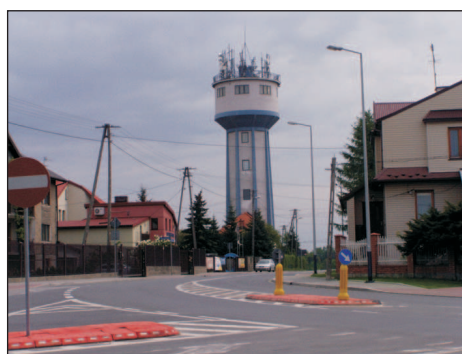
Phot. 25. Tower water reservoir in Kraków - the district of Skotniki (photo: J. Pawełek)
