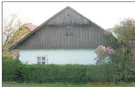
Phot. 49. A house plastered with clay and whitewashed with lime and some addition of ultramarine: the gable with a double overhang, finished up with a decorative element; a hedge separates the house from the road (photo: P. Herbut)
