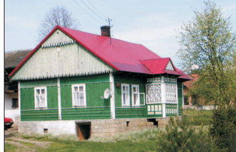
Phot. 63. A house from 1900, on an underpinning, with a closed porch: window frames, corners, slats covering clapboard contact points are painted white and strongly contrast with green walls (photo: P. Herbut)
