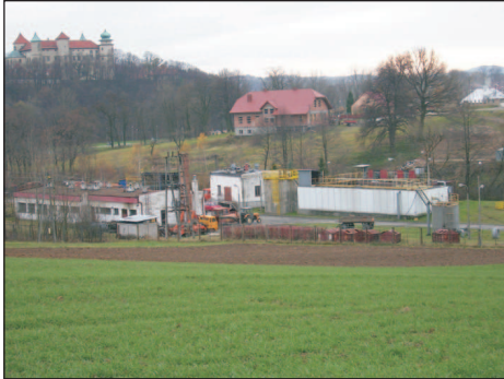
Phot. 26. Sewage treatment plant in Nowy Wiśnicz (photo: G. Rudek)
