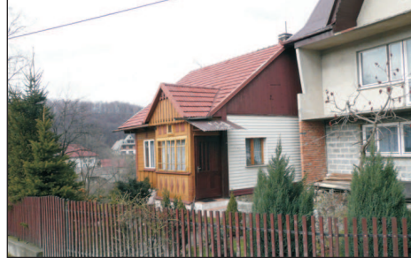
Phot. 67. A house with a beautiful porch, partially taken down to make space for a new building (photo: W. Bieda)
