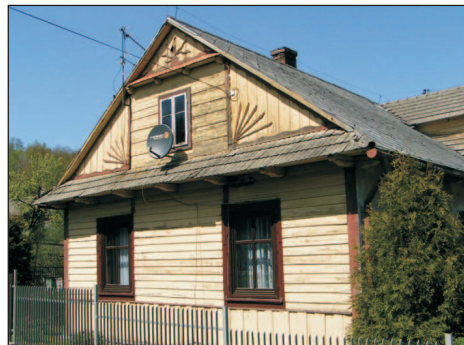
Phot. 61. A gable with two small roofs: a carved slat running along the eaves and a radial ornament - elements typical for the architecture of the Podhale region. New windows on the ground floor correspond to traditional patterns (photo: P. Herbut)
