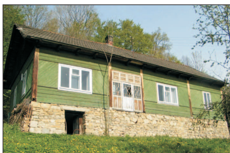
Phot. 46. A house on a plot with southern orientation situated parallel to contour lines: high stone underpinning; an entrance to the cellar with a stone vault; walls covered with clapboards; new windows differ from typical windows for that region in terms of size and structure; the glazed surface of the entrance hall with decorative shapes and panels (photo: P. Herbut)
