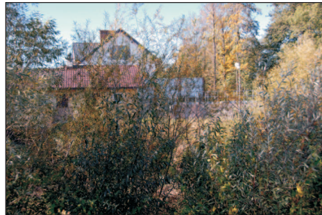
Phot. 38. Sewage treatment plant in Wiśniowa seen from the road (photo: G. Kaczor)
