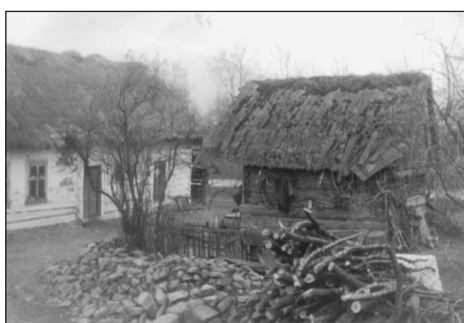
Phot. 42. The year 1970, Na Sodku, the oldest farm in Wiśniowa; a house and a building for livestock with double-pitched thatched roofs (from the Kronika Szkoły Podstawowej w Wiśniowej of 1970)
