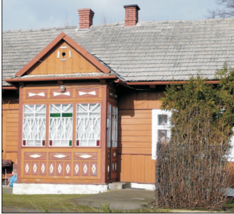
Phot. 58. A closed porch: apart from the porch windows decoratively divided into smaller sections and planks covered with patterns on the walls, coloured panes preserved to this day in the upper and bottom part of the transom window, very popular in the past; the tympanum of the porch with an opening and a small roof separated from the wall (photo: W. Bieda)
