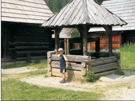
Phot. 15. Well with a wooden case (photo: G. Kaczor)
