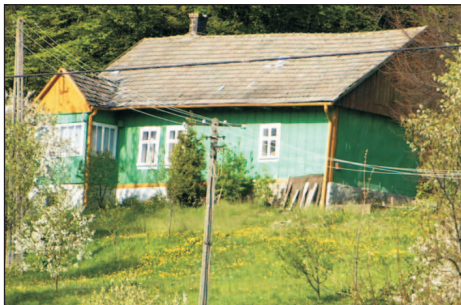
Phot. 64. A house with a closed porch, situated on the side: green walls, white window frames, while the corners; the ground beam, and the tympanum of the porch are painted light brown (photo: P. Herbut)
