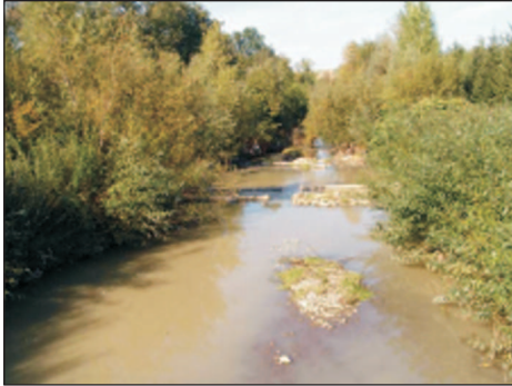
Phot. 78. Lower part of the Krzyworzeka river with river regulation structures (photo: K. Boroń)
